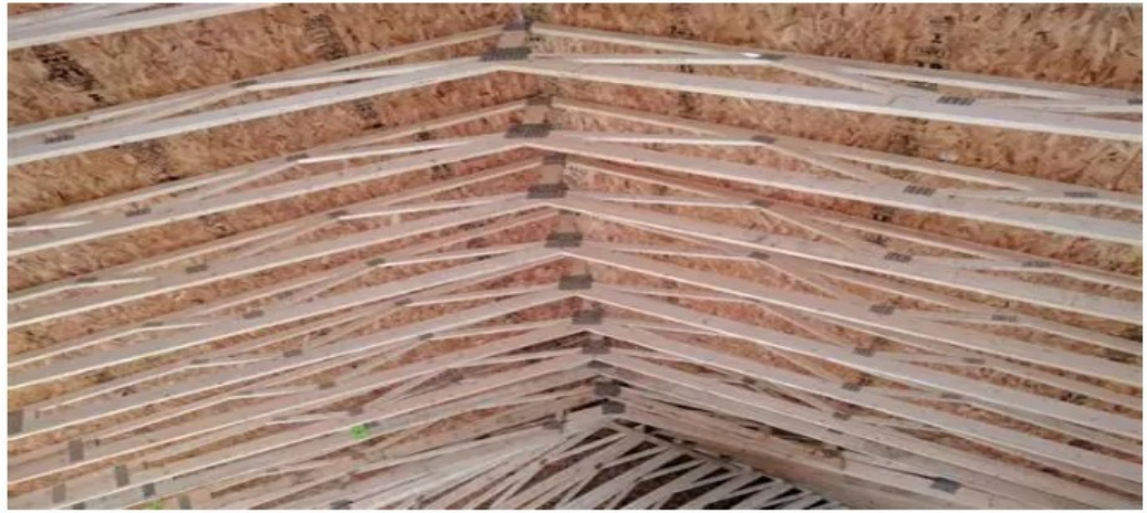
Parallel Chord Wood Truss
